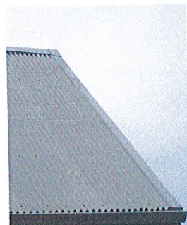
1 - CORRUGATED METAL ROOFING
