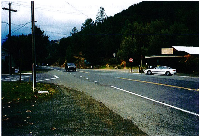
Intersection of Highway 29/Lincoln Avenue, Silverado Trail and Lake Street
