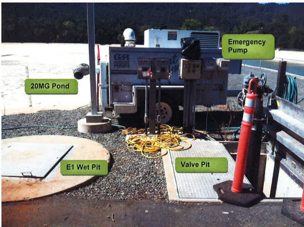
39 Photo 1 - E1 Wet Pit Valve and 20MG Pond
