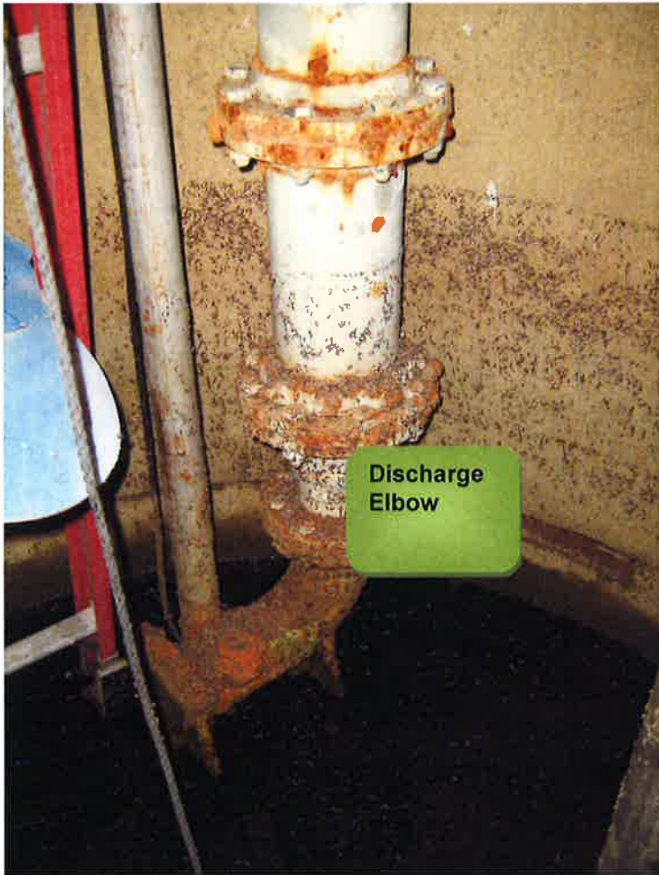
Photo 3 – Discharge Elbow Corrosion
