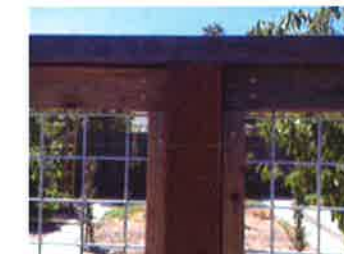
WOOD FENCE W/ HOGWIRE PANELS DETAIL
