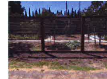
WOOD FENCE W/ HOGWIRE PANELS 4' AND 8' HEIGHTS
