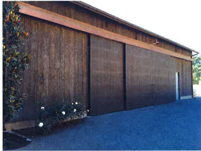
SURFACE TRACK SLIDING DOORS WITH COPPER LIGHT ABOVE
