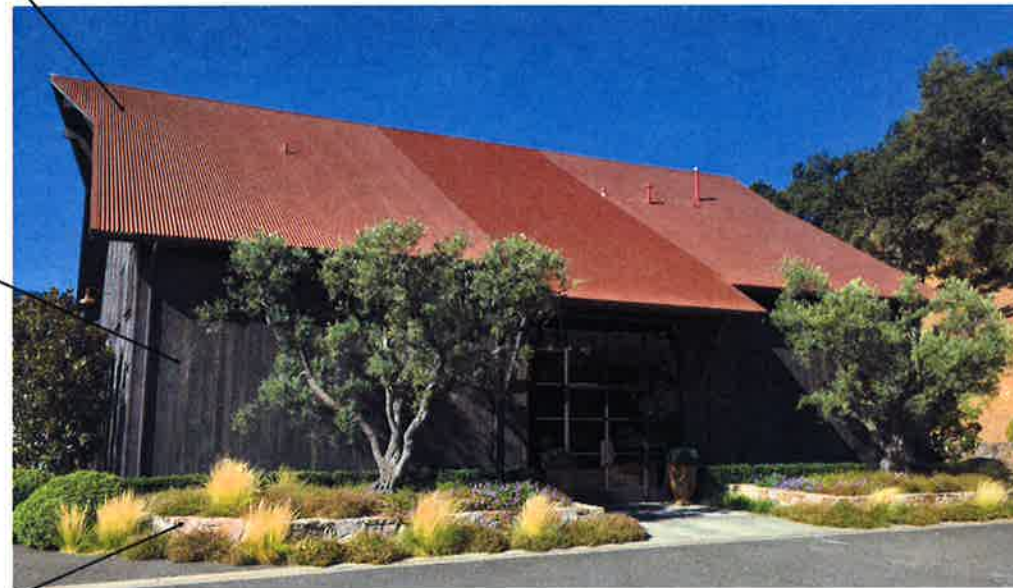
PHOTOGRAPH AT THE EXISTING FRONT ENTRY. EXTERIOR FINISHES AT ADDITION TO MATCH CURRENT MATERIALS.
