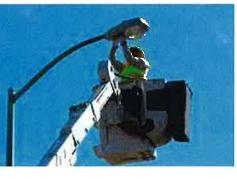
As part of our commitment to provide customers with safe, reliable, affordable and clean energy, Pacific Gas and Electric Company (PG&E) is upgrading its non-decorative, high pressure sodium vapor (HPSV) streetlights with more energy-efficient, light-emitting diode (LED) fixtures.
