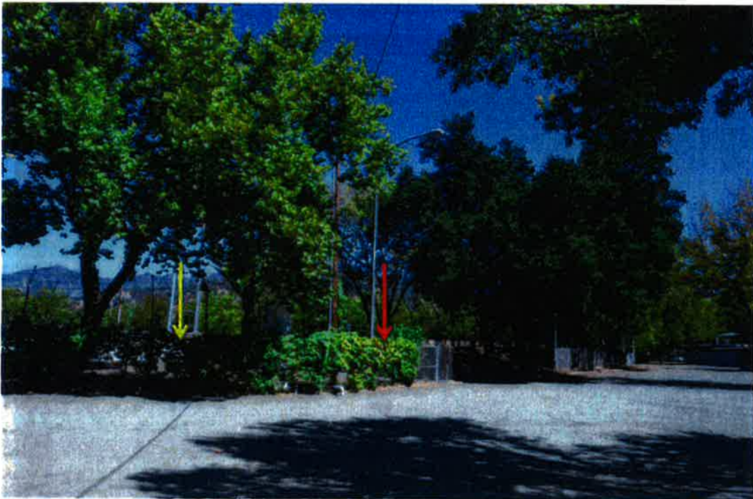
Arrow indicates suggested alternative equipment shelter location to right of tree #3 near access road gate (red arrow). Yellow arrow indicates current shelter location.
