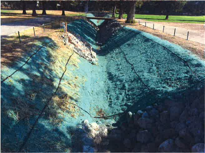
GRANT STREET STORM DRAIN – PHASE II
