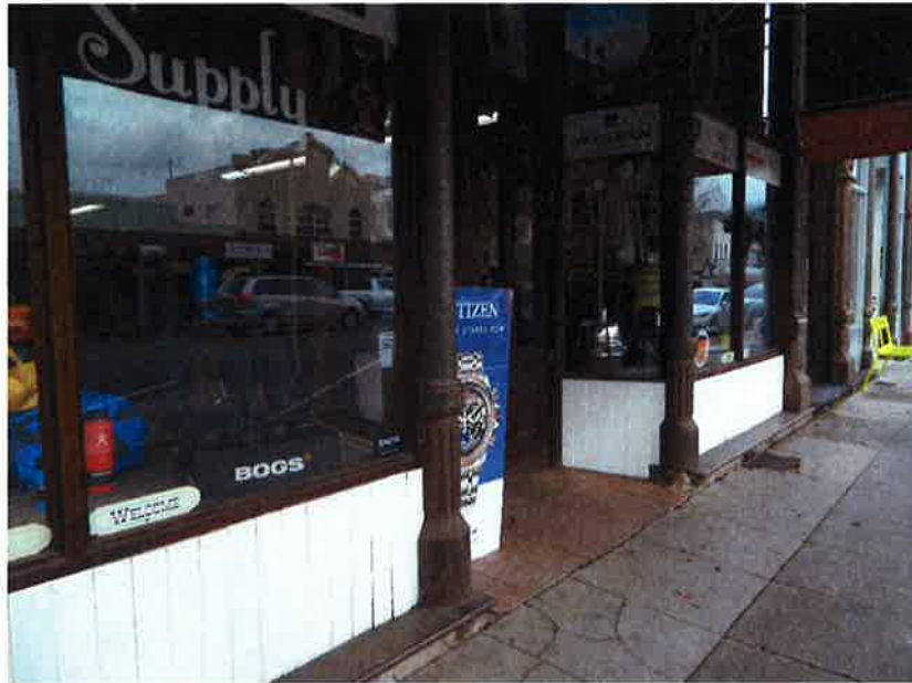
Figure 26. First Story, storefront with cast-iron columns.
