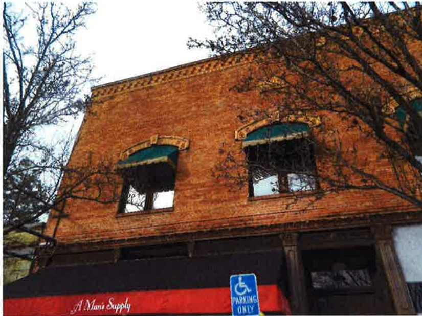
Figure 30. Second Story showing the cornice and widow crown details.
