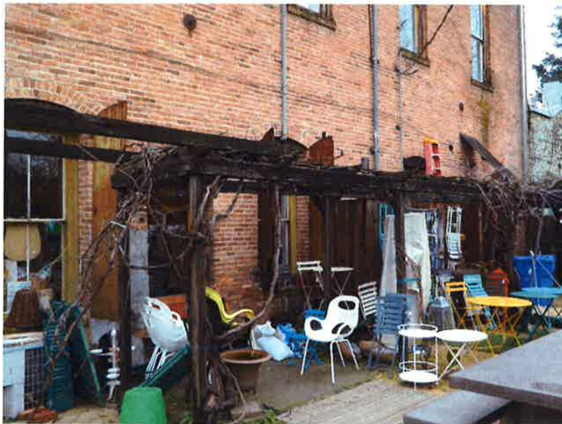
Figure 33. West Elevation, showing the iron shutters.
