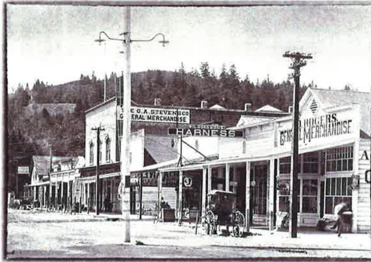
Figure 7. ca. 1905, showing the C.A. Stevens General Merchandise signage on the Odd Fellows Hall.
