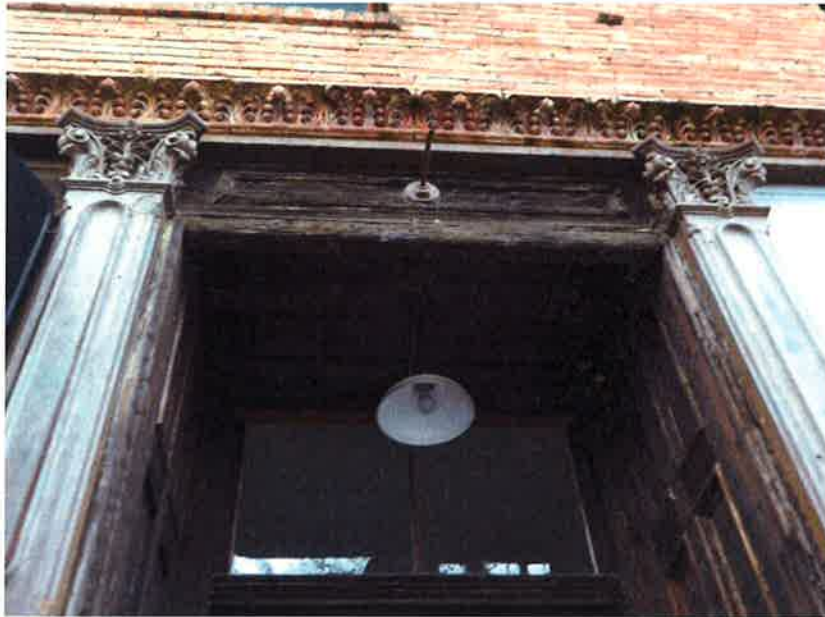
Figure 29. Corinthian pilasters at the centered second floor entry.
