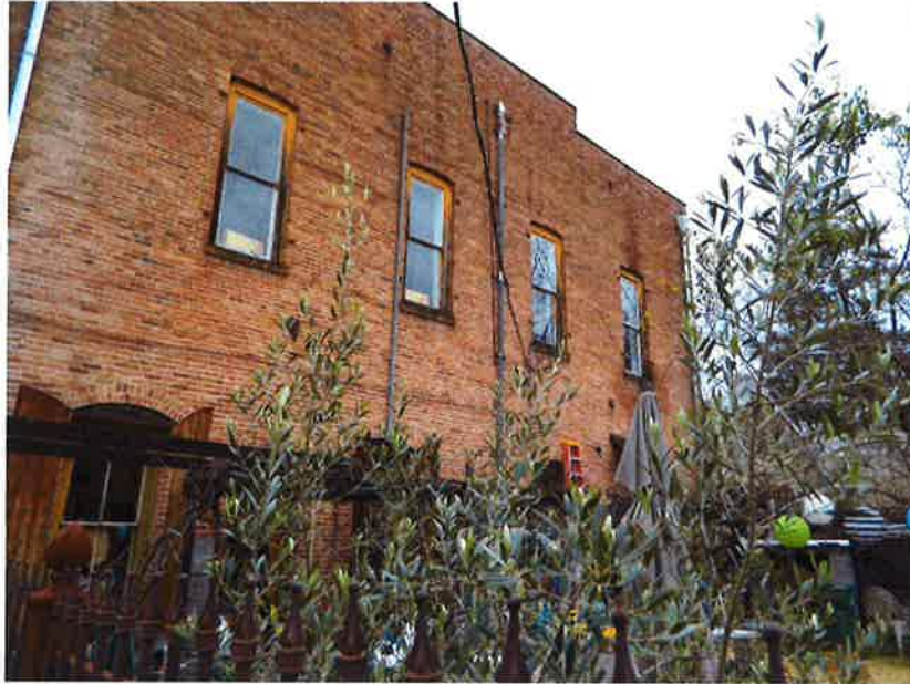
Figure 32. West elevation, facing south.
