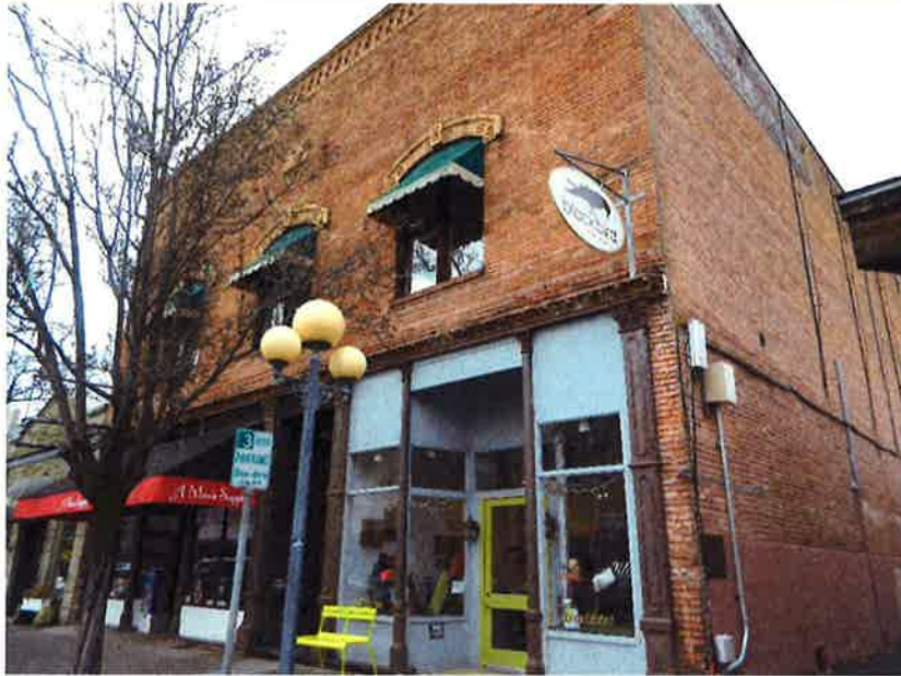
Figure 28. The retail boutique storefront, facing southwest.
