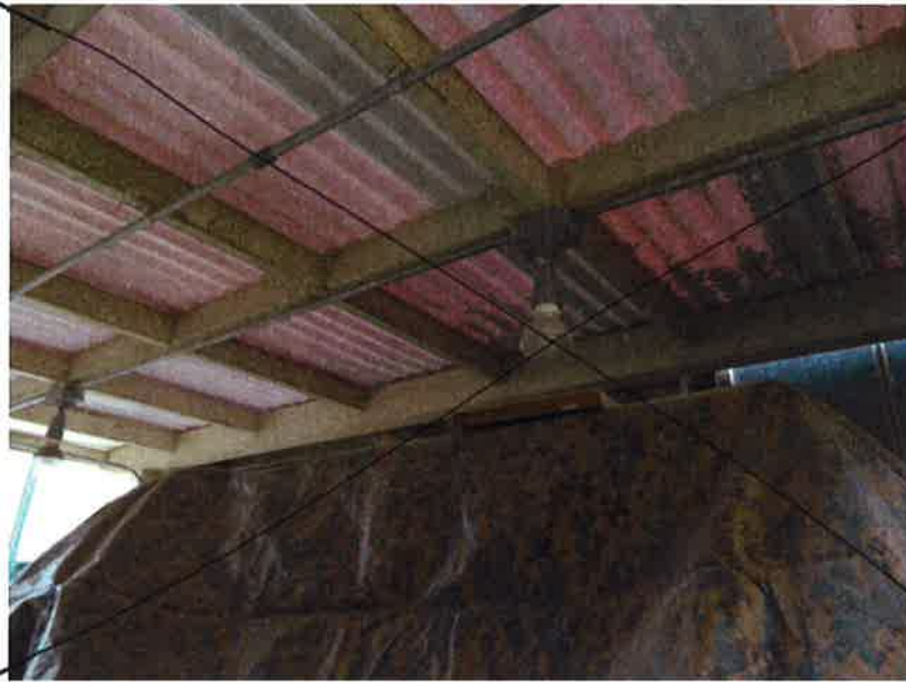
Figure 24. Corrugated, plastic awning at the rear of the building.
