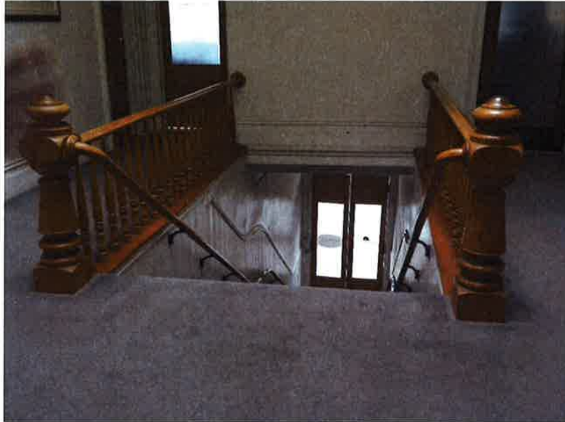
Figure 35. Interior second floor, showing the first story main entry doors.
