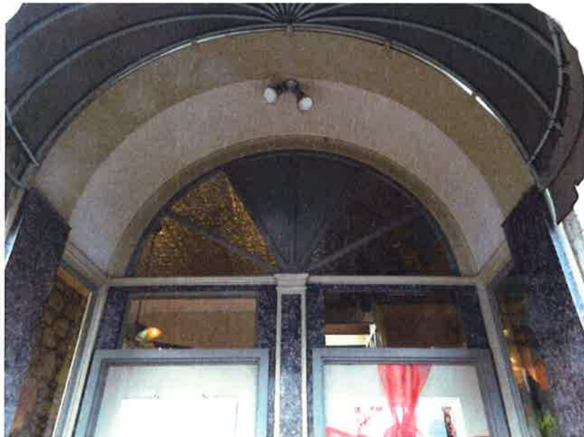
Figure 11. The fanlight and transom windows within the recessed arched entryway.
