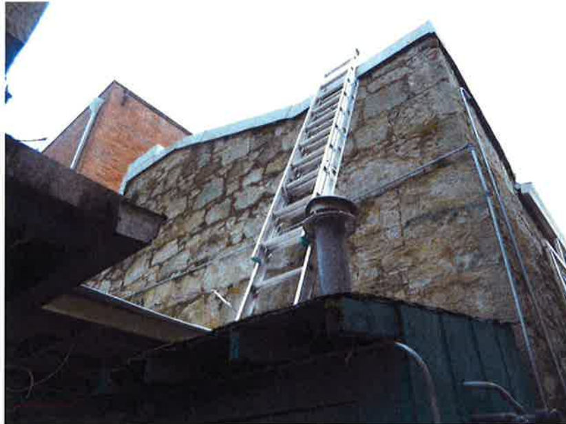
Figure 15. West Elevation, facing northeast.
