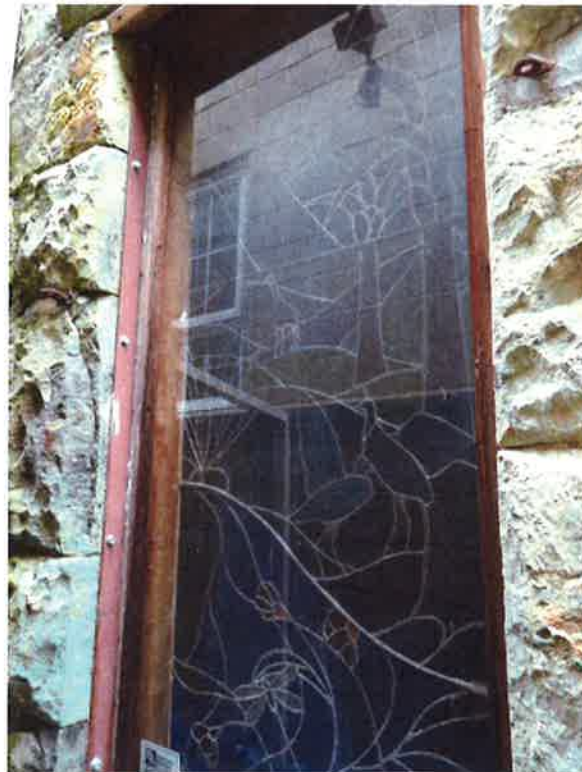
Figure 14. Modern Stain glass window set within the original window opening.
