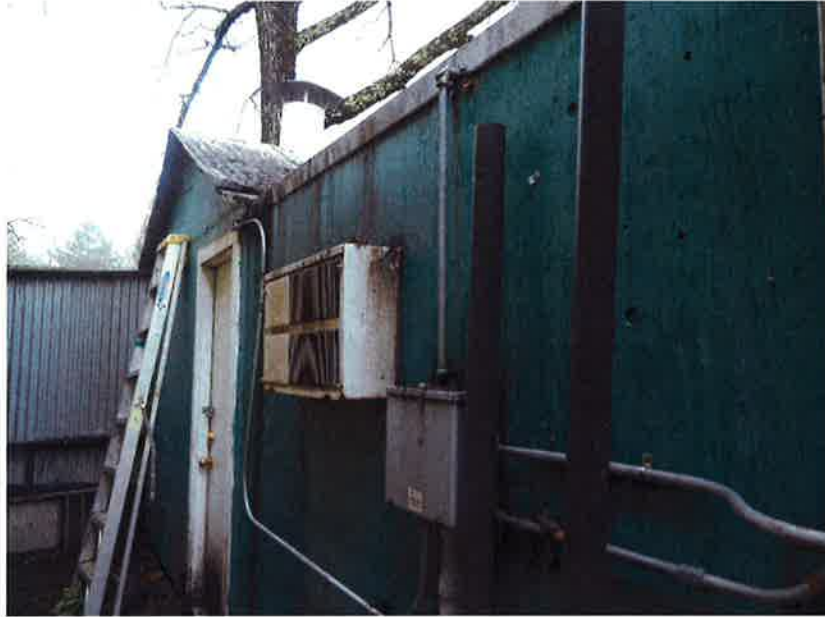
Figure 23. Sheds, at the rear of the property, facing northwest
