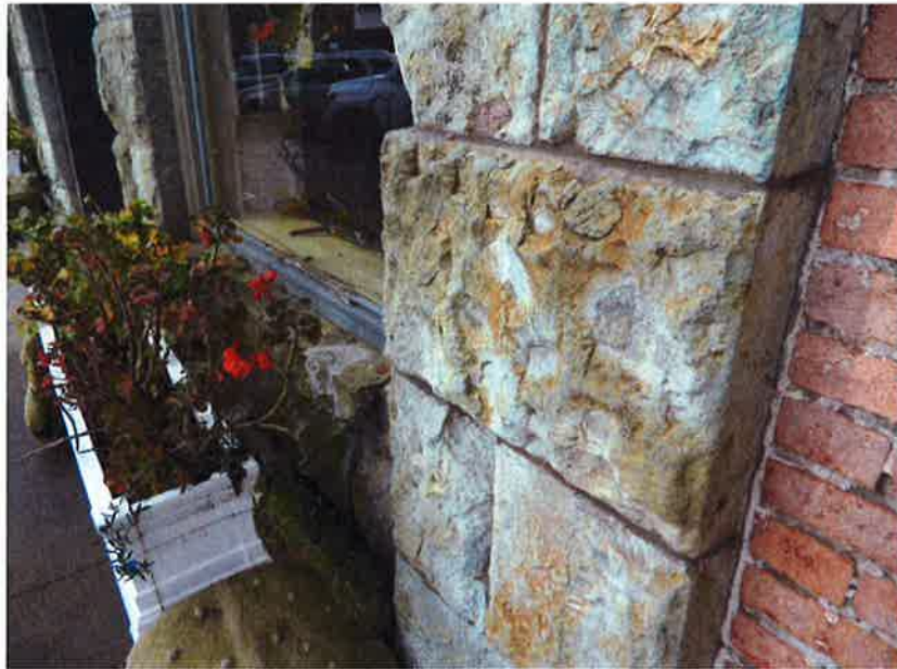
Figure 9. Rough-cut course stone details on the east elevation.
