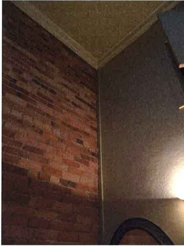
Figure 20. Interior of C.A. Stevens showing the shared interior wall.
