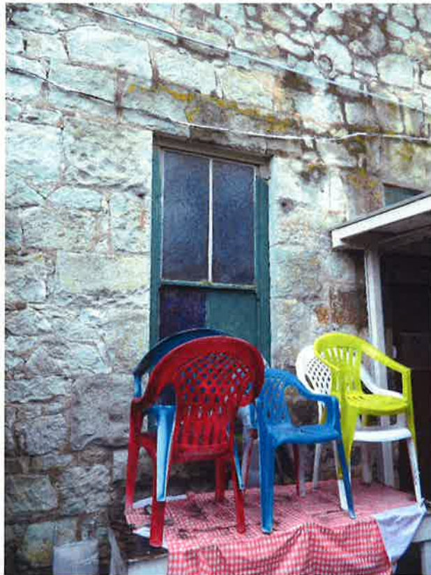
Figure 17. Double-hung wood window.
