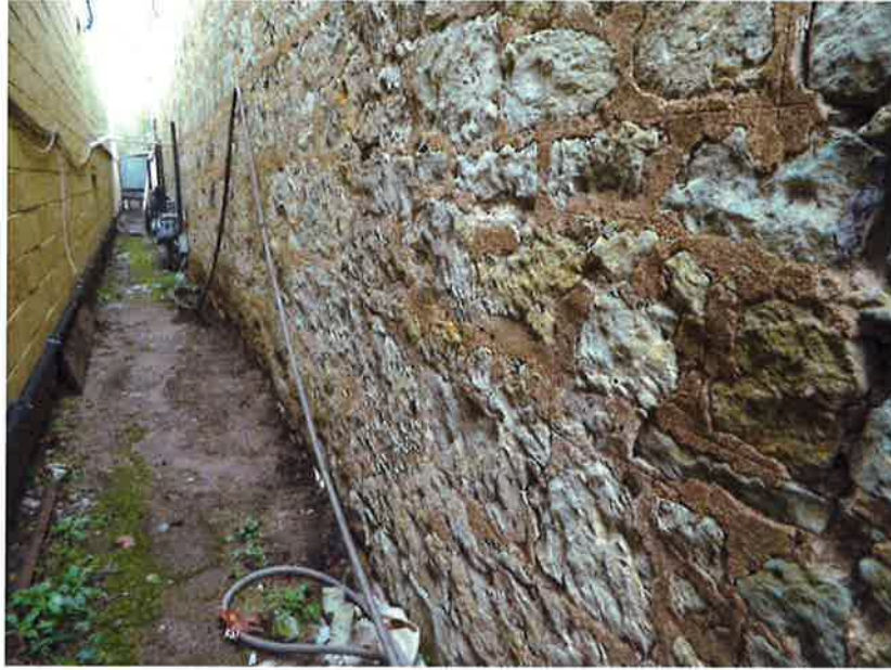
Figure 12. Rough cut stone along the south elevation.
