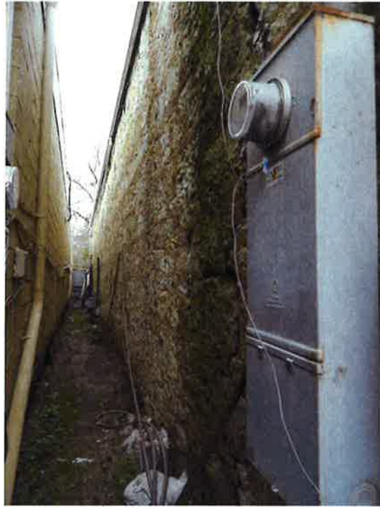
Figure 13. South elevation, facing west.
