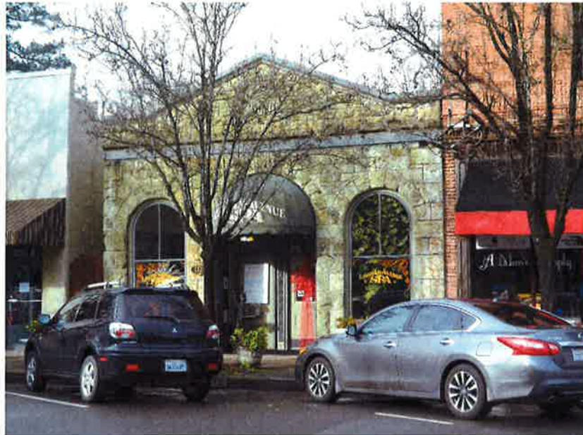
Figure 8. East Elevation, facing southwest.
