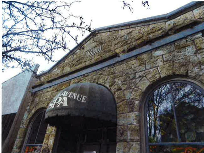
Figure 10. East elevation, facing southwest.
