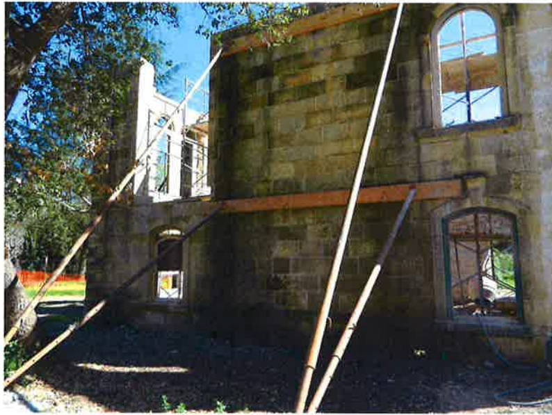
Figure 8: North elevation, facing south.
