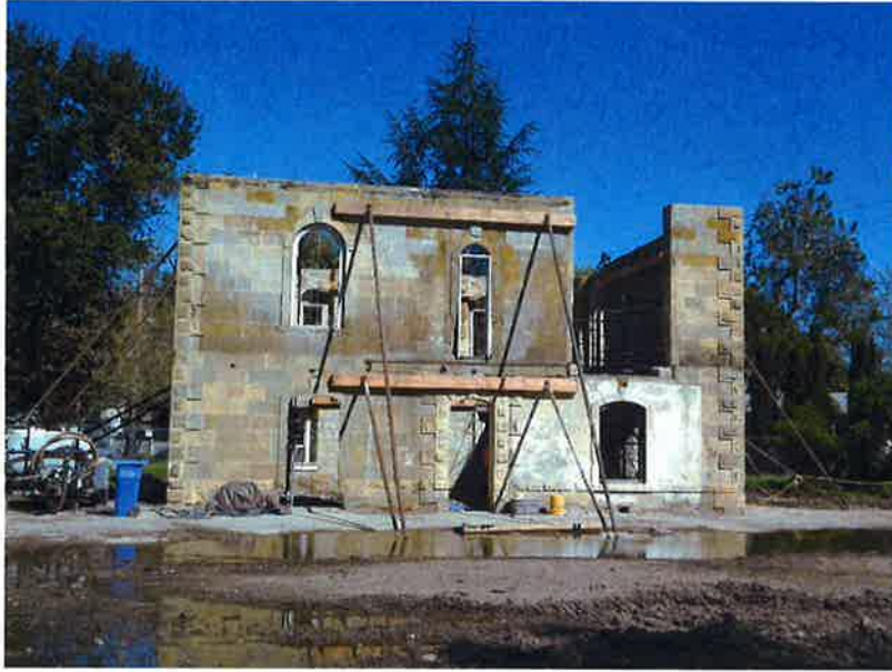
Figure 7: West elevation, facing east.
