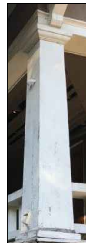
ORIGINAL TAPERED PORCH COLUMN
