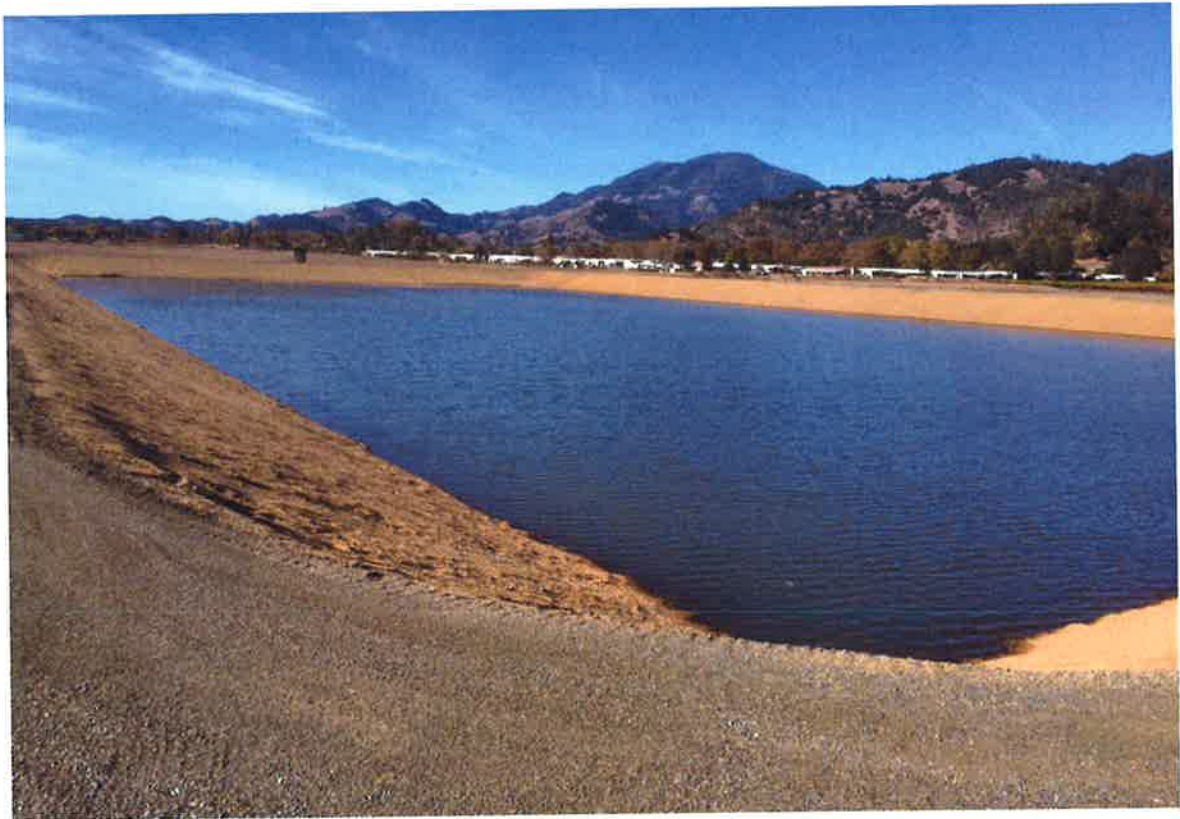
RECYCLE WATER POND
