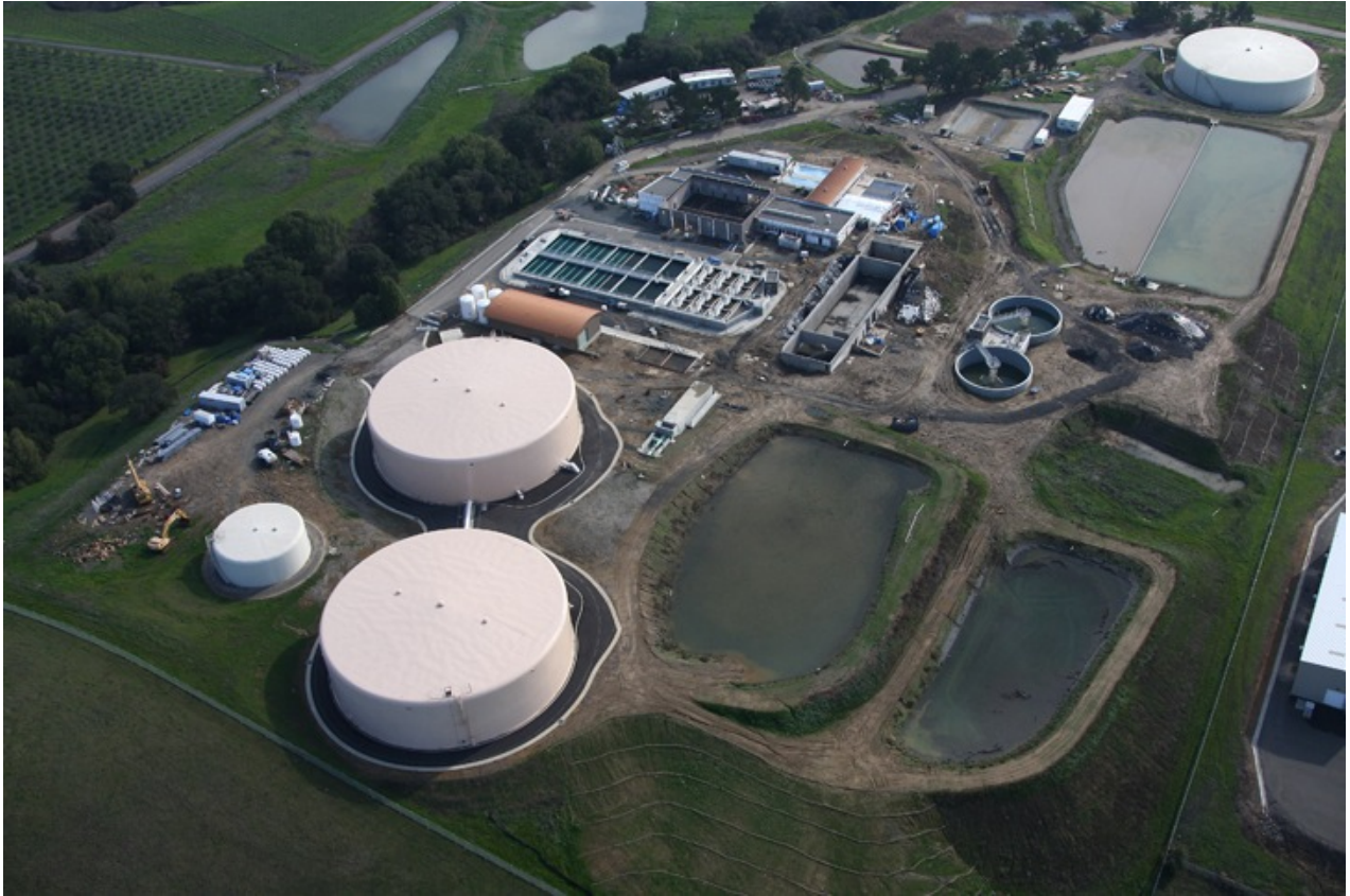
Jamieson Water Treatment Plant aerial view.
