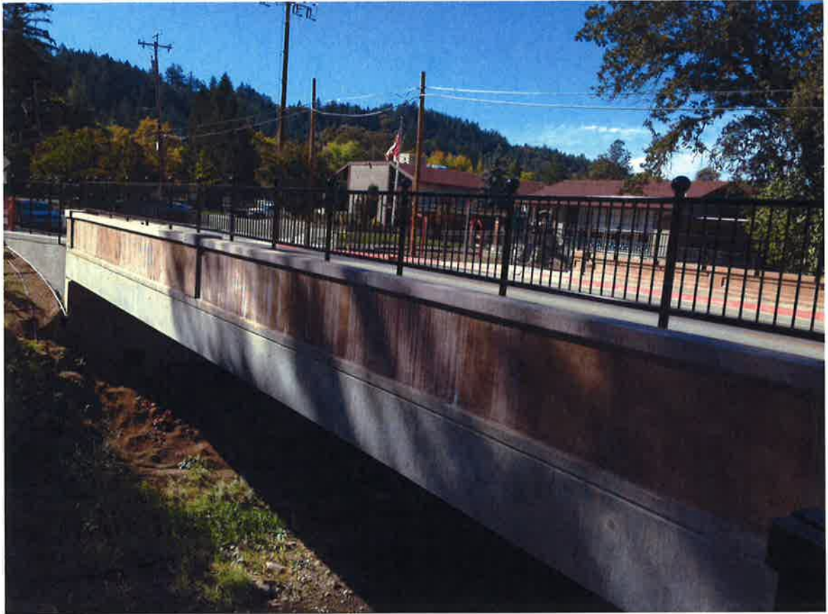
BERRY STREET BRIDGE
