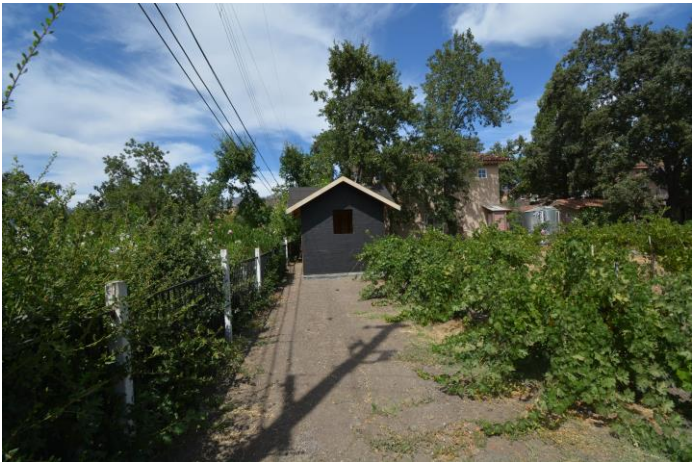
New PG&E Utility Shed
