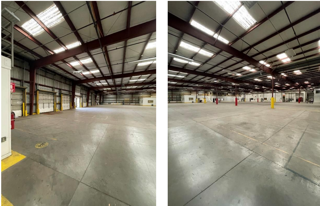
79 View of storage facility facing north – west & east views.
