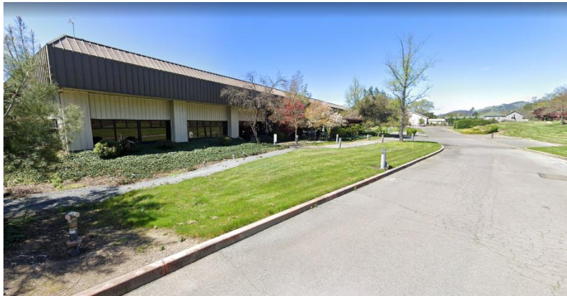
View of parking lot & front of building looking west.
