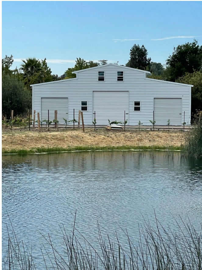
Photo 8: Metal building adjacent to pond
