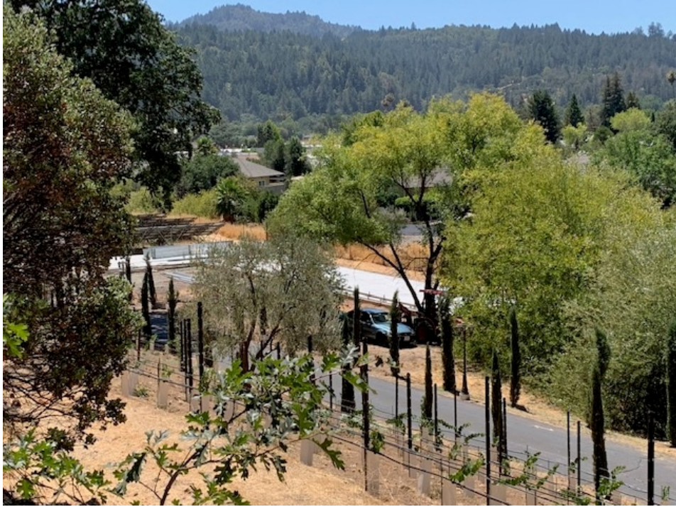
Photo 7: Large foundation/slabs – Red Tagged
