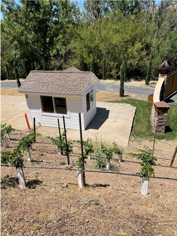
Photo 1 &2: Entrance gate & storage shed on (E) concrete slab
