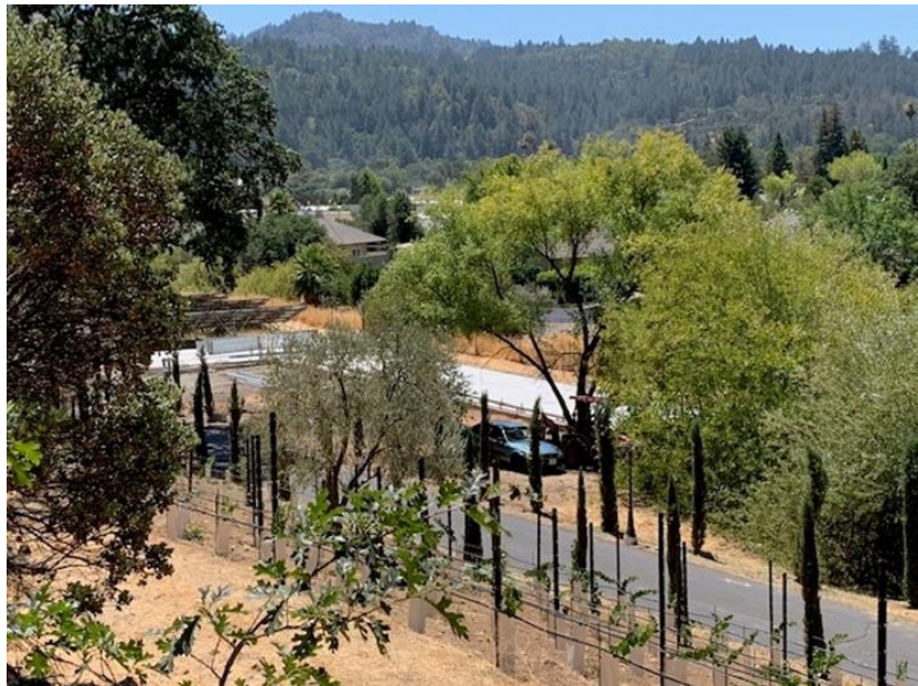
140 Unpermitted Garage Pads
