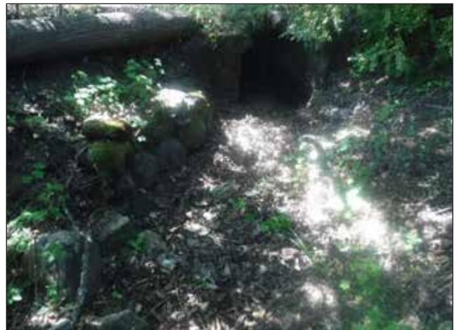
**PHOTO 6:** 3'x3' arch culvert under driveway
