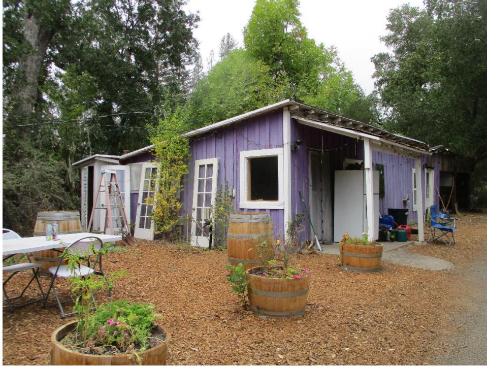
Figure 14. Photograph showing the converted addition, facing northeast.
