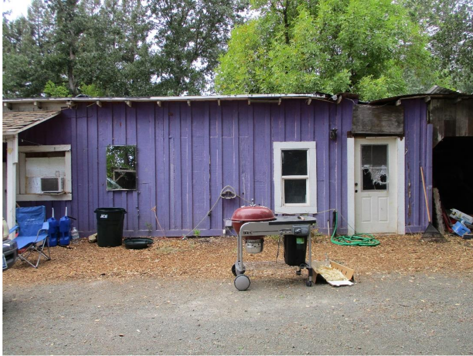
Figure 16. Photograph showing the secondary entrance to the building, facing north.
