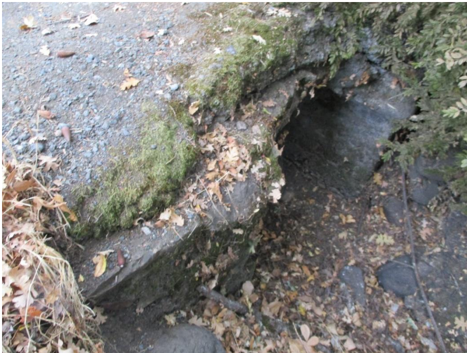
Figure 12. Photograph showing the concrete abutments and stone piers.
