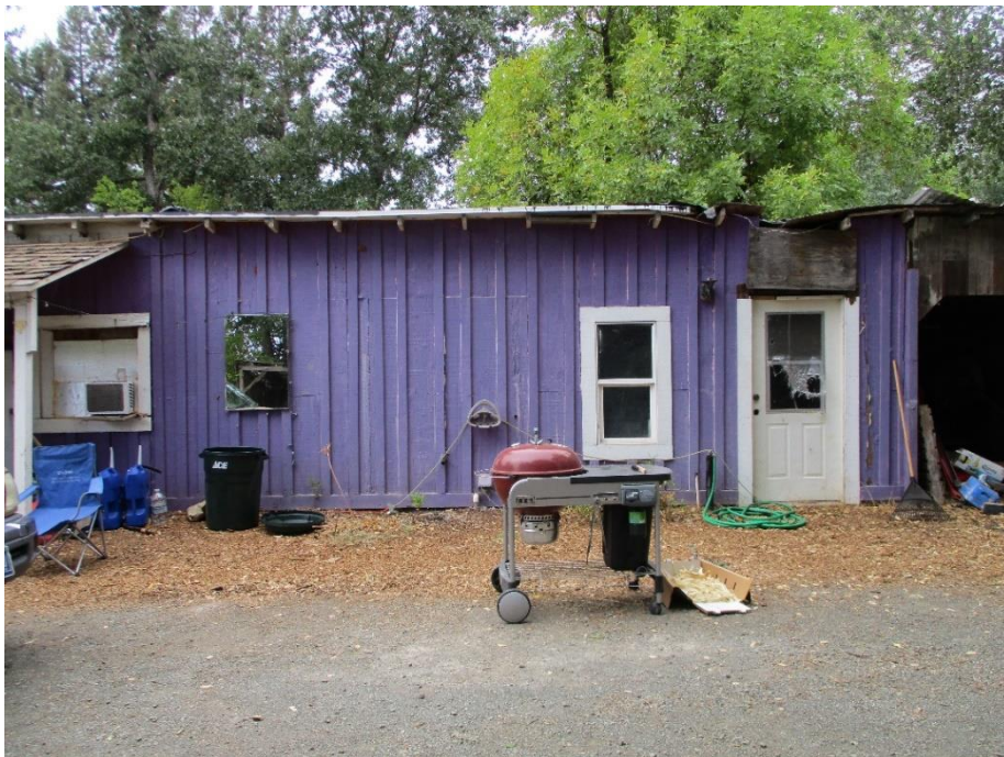
Figure 2. Photograph showing the secondary entrance to the building, facing north.
