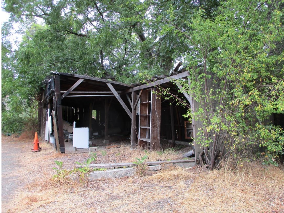
Figure 21. West elevation, facing east.
