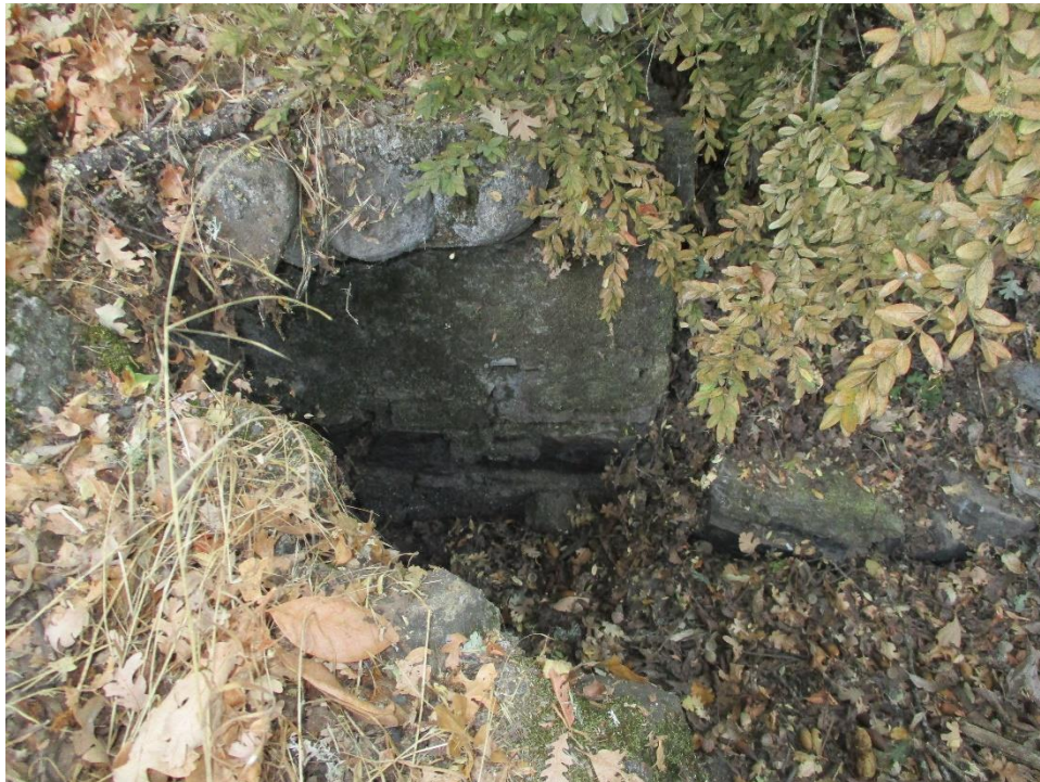
Figure 27. Photograph showing the arched opening of the ca. 1920 stone bridge.
