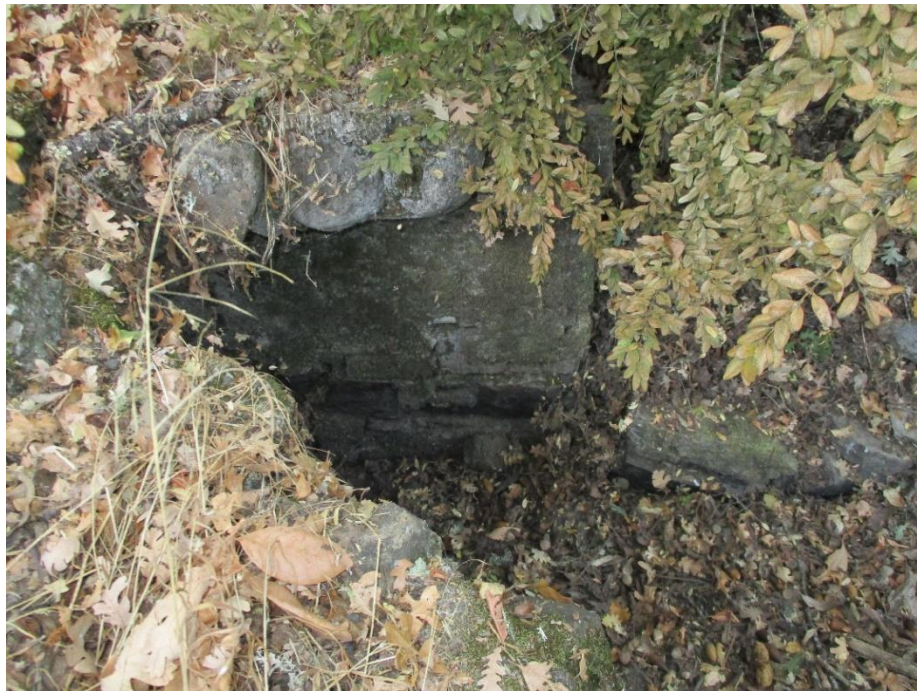
Figure 13. Photograph showing the arched opening of the ca. 1920 stone bridge.
