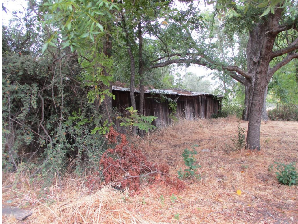
Figure 23. South elevation, facing northeast.
