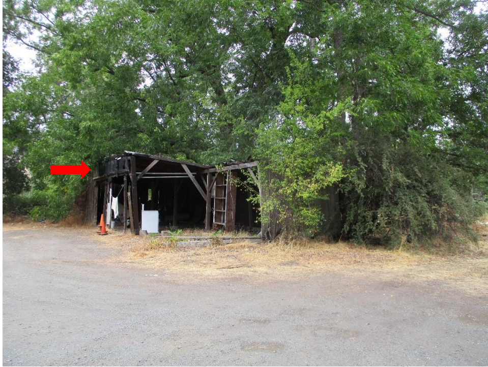
Figure 20. Photograph showing the northwest corner of the ca. 1950 barn, with fire damage along the shed roof (red arrow), facing east.
