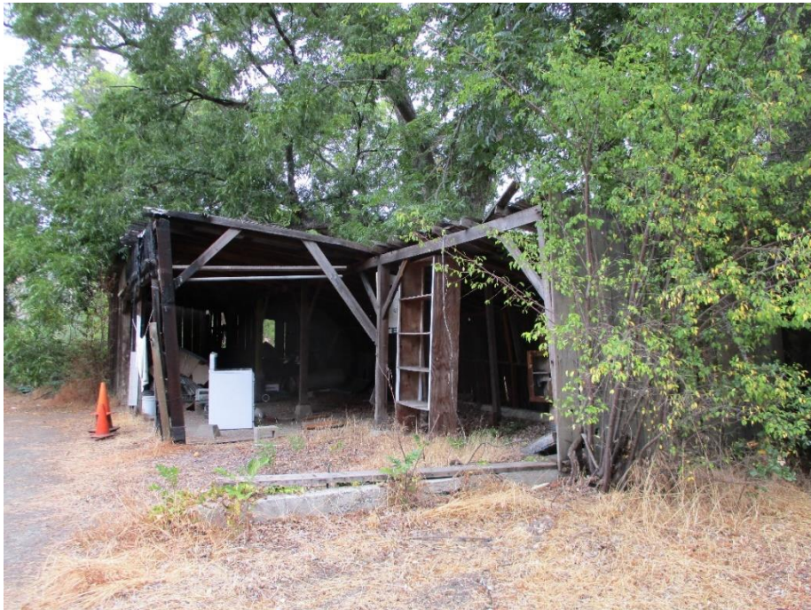
Figure 7. West elevation, facing east.
