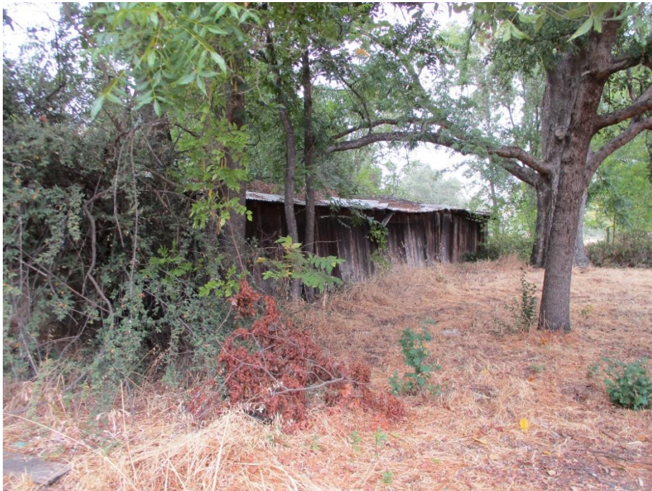
Figure 9. South elevation, facing northeast.
