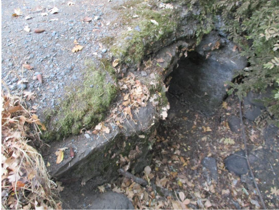
Figure 26. Photograph showing the concrete abutments and stone piers.
