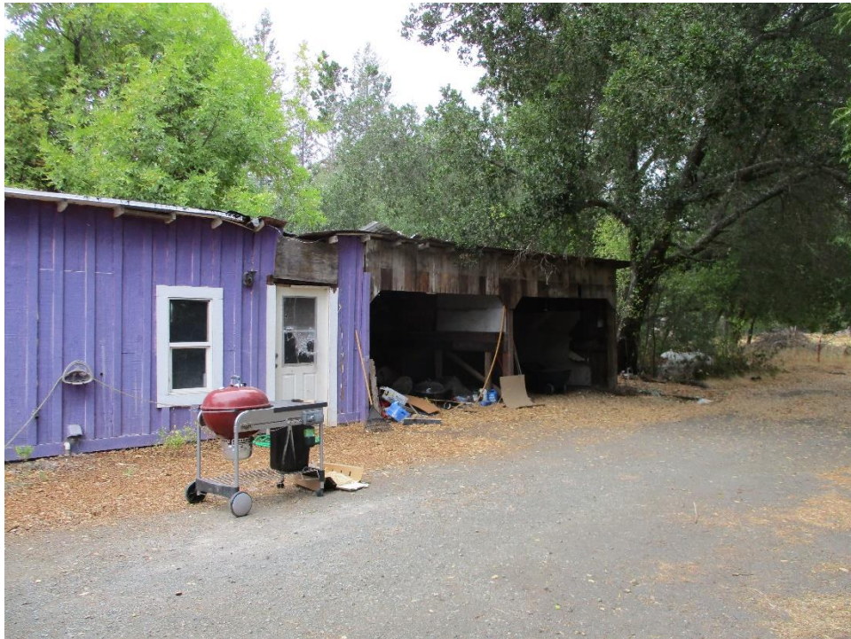
Figure 17. Photograph showing the original section with the two bay openings facing northeast.
