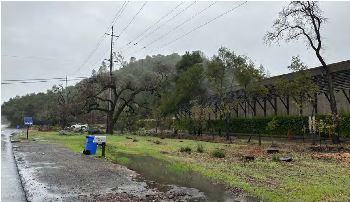
Figure 3.1-2. Proposed Rutherford Pump Station Site
