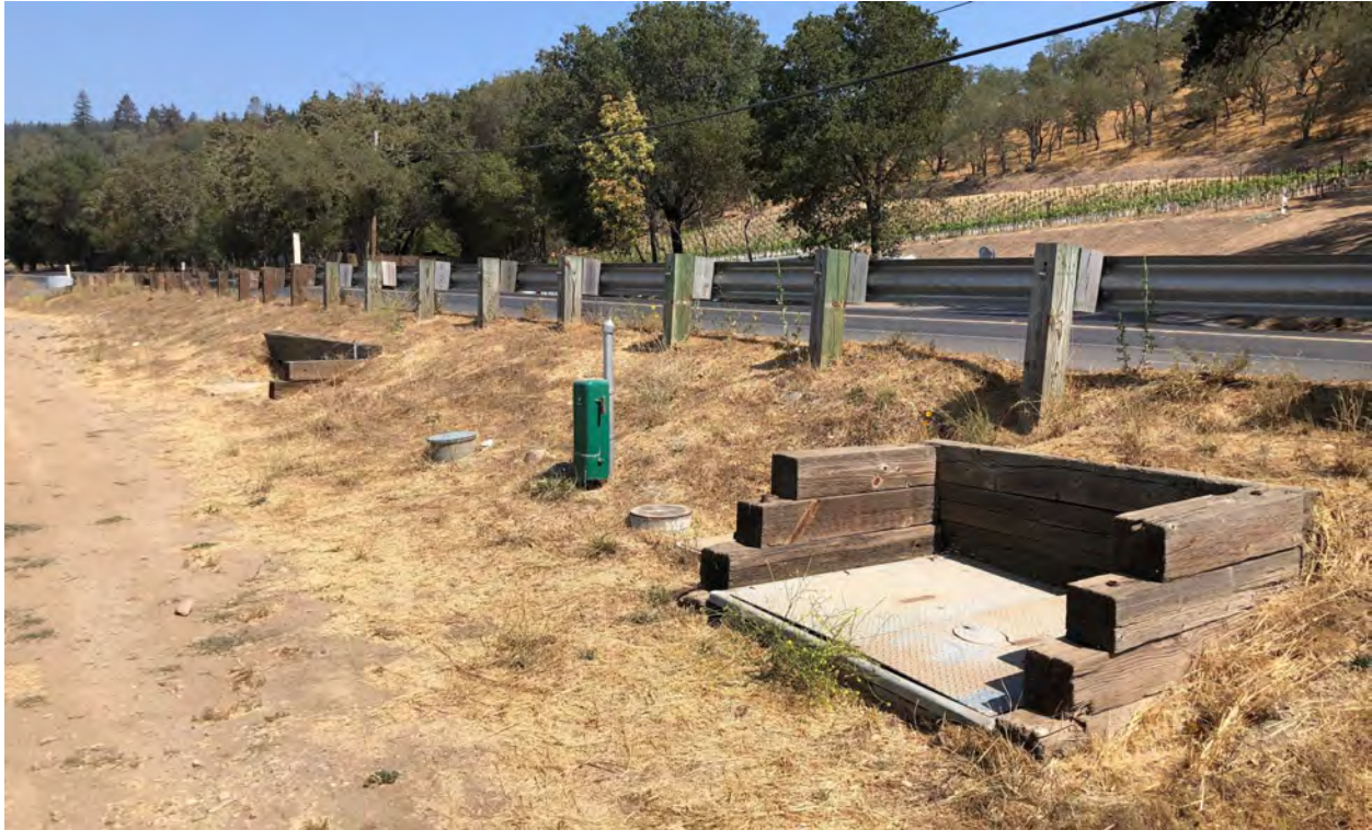
Figure 2-5. Photo of the Napa Meter Location
