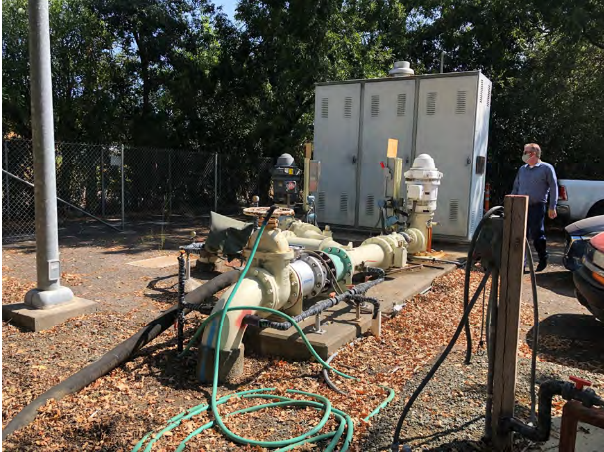
Figure 3.1-1. Dunaweal Pump Station Site
