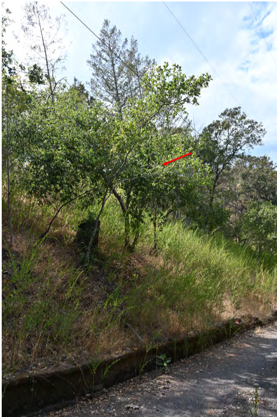
Tree #1, a coast live oak located in future road turnout. Located below electrical distribution lines and subject to clearance pruning.
