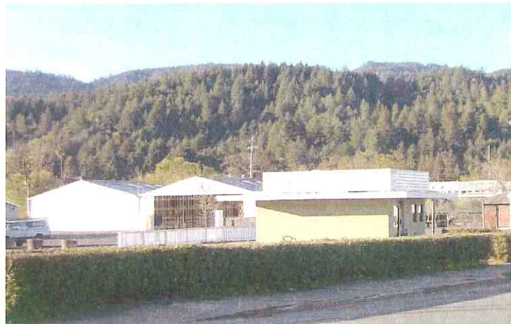
Image 11C. Post construction, photo rendition of hillside upon project completion
