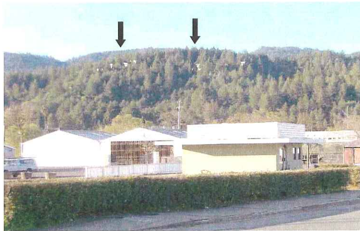
Image 11B. During construction, white areas illustrate temporary construction sites
