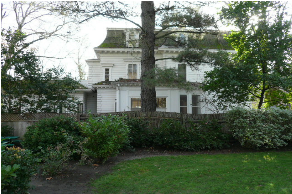
West side elevation of house from Pioneer Park. "Notch" at left to be filled in with small addition. Fence in foreground to be replaced
