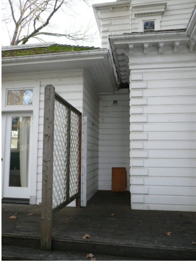
“Notch” to be filled in by new addition. Lattice fence to be removed
