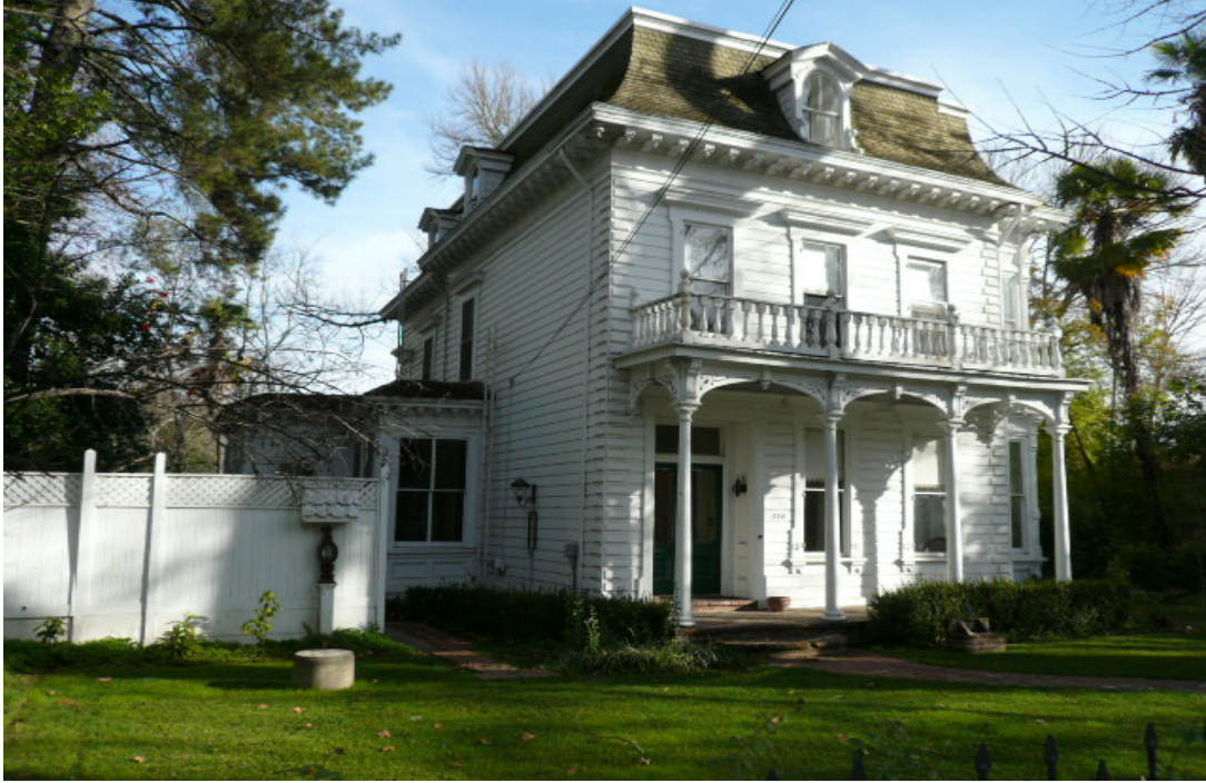
Front elevation from near Pioneer Park. Fence at left will be replaced with similar fence moved toward rear, to line up with dining room window on left of house
