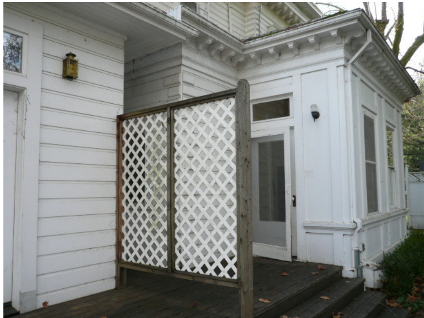
View of area where small addition will be located (east elevation)
