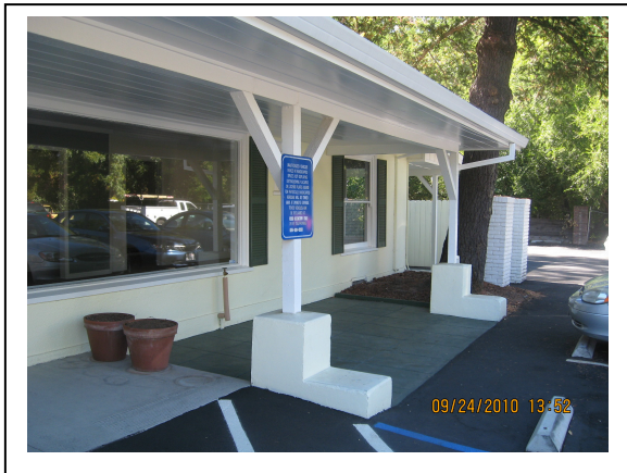
59 (P) 1307-A, Outdoor Patio Seating near Front Entry
