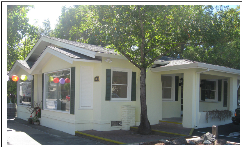
[Photo] View of Store Frontage along Lincoln Avenue
